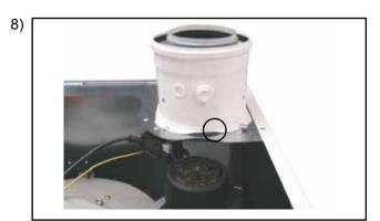
After removing the upper casing cover, undo the self-tapping screw at the balanced flue locking mechanism.
