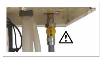
Fig.: Gas connection Escaping gas may cause poisoning or an explosion
