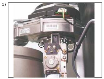
Unscrew the mixing chamber from the fan (three Allen screws 5 mm), and remove air inlet pipe if necessary
