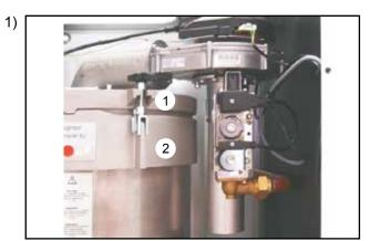
Unplug the connector  ${\Large \textcircled{1}}{\Large \textcircled{2}}$  (first unscrew the Phillips head screws)
