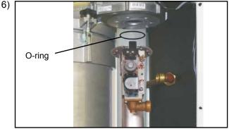
After assembly of the gas restrictor, gas combination valve and air inlet pipe, push the O-ring lubricated with silicone grease into the packing groove of the fan and refit the mixing chamber.
