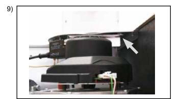
Slide the balanced flue locking mechanism in the direction of the arrow. Pull the flue pipe up out of the condensate pan.
