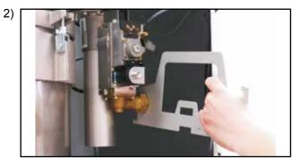
Undo gas connection at the gas combination valve
