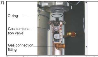
Push the O-ring, lubricated with silicone grease, into the packing groove of the fan and fit the mixing chamber with the gas combination valve to the burner fan.
