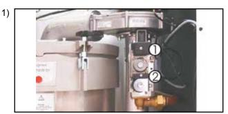
Unplug the connector @@ (first unscrew the Phillips head screws)
