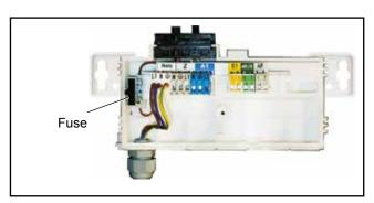
Fig.: Terminal box cover open
