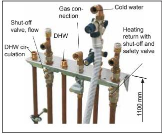
Fig.: Connection to concealed mounting bracket for surface mounting (accessory)
