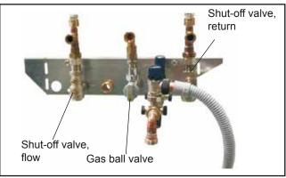
Fig.: Shut-off systems at concealed mounting bracket for flush mounting (accessory)
