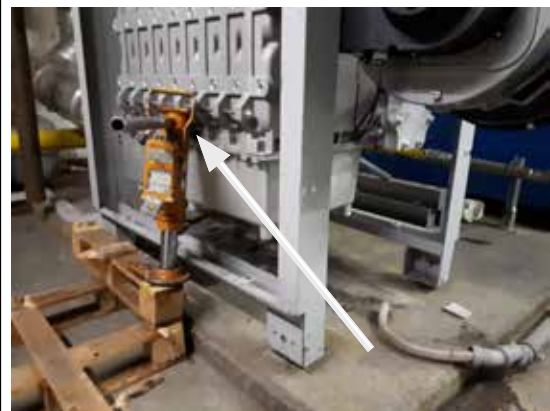
Jack beneath connecting rod
