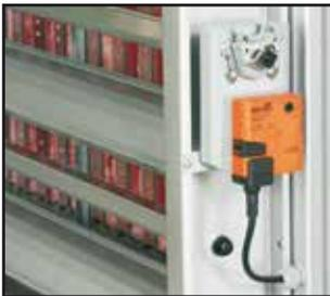
Check that the dampers and linkage move freely.
